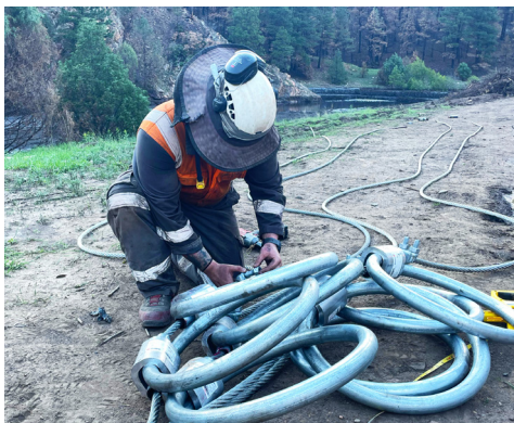
Debris Flow Barrier Construction Plimmerton, New Zealand
